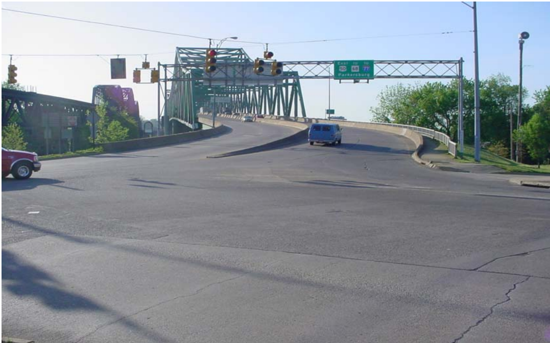
Pictures of the Belpre Bridge Intersection.
