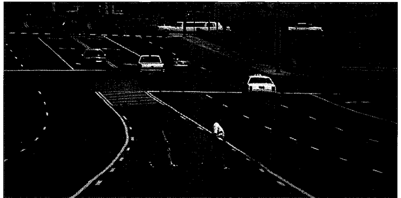
FIGURE 1-5. Medians can greatly improve conditions for pedestrians on wide, multi-lane arterial streets.
