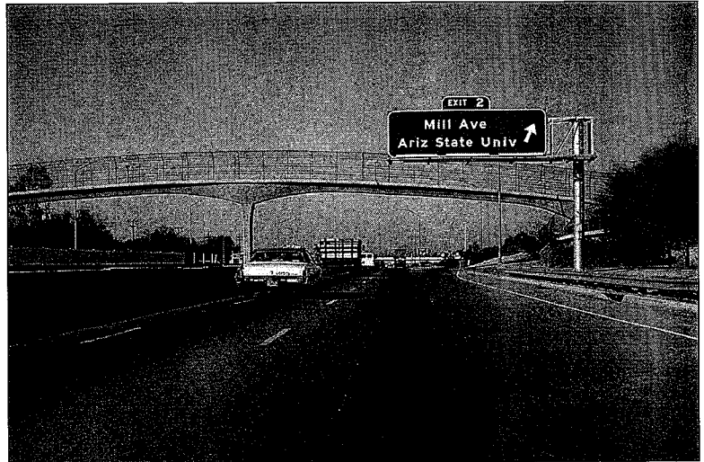
FIGURE 10-1. Pedestrian overpasses and bridges are often needed for high-speed or heavily travelled roadways.
