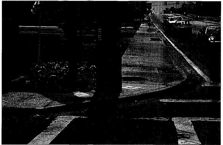
FIGURE 3-7(a). Sidewalks should be clear of poles and other objects.
