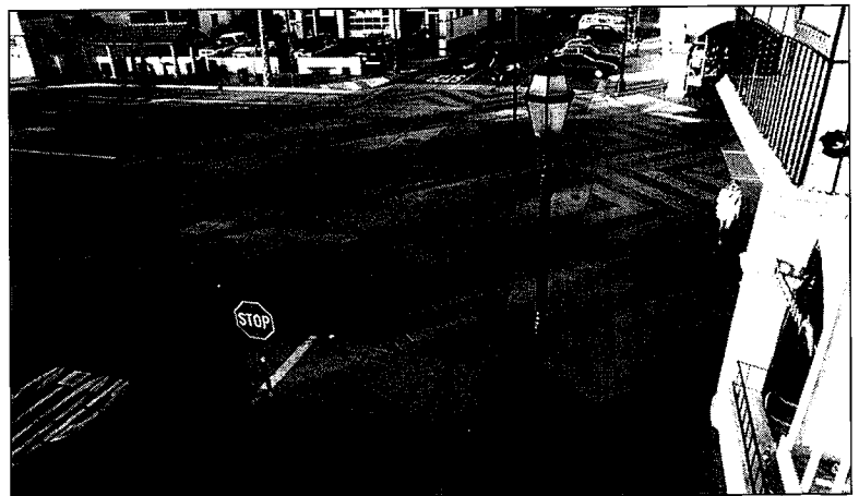
FIGURE 12-10. Raised intersections can enhance pedestrian safety by reducing traffic speeds.
