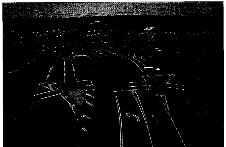
FIGURE 1-9. Properly designed right-turn slip lanes with pedestrian refuge islands can enhance crossings for pedestrians.
