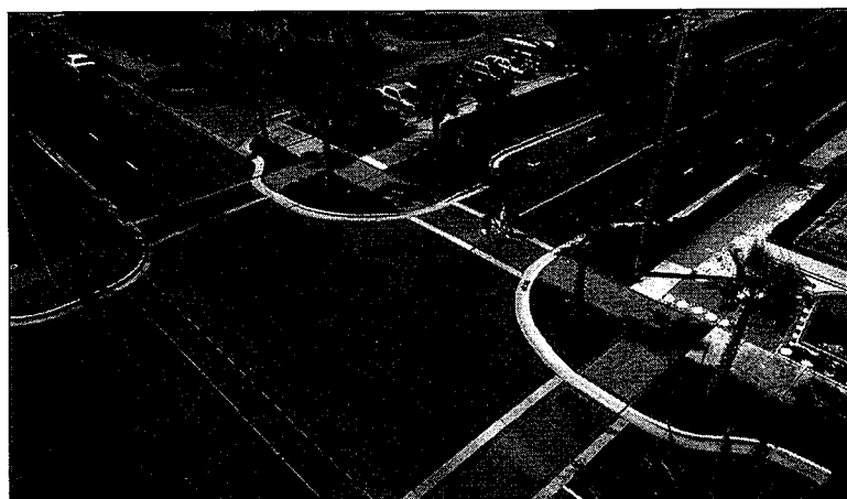
FIGURE 12-7. Streets narrowed at the crosswalk reduce the pedestrian exposure to vehicular traffic.
