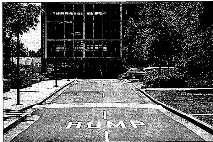
FIGURE 12-9. Speed humps reduce traffic speeds to about 20 to 25 mph.
