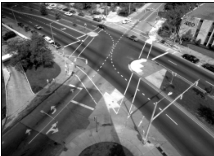
Figure 11-4. This intersection could be improved in many ways. Note that pedestrians leaving the lower right corner must walk a distance of over 20 feet just to get to the first lane to be crossed—a channelized slip lane would reduce this distance.
