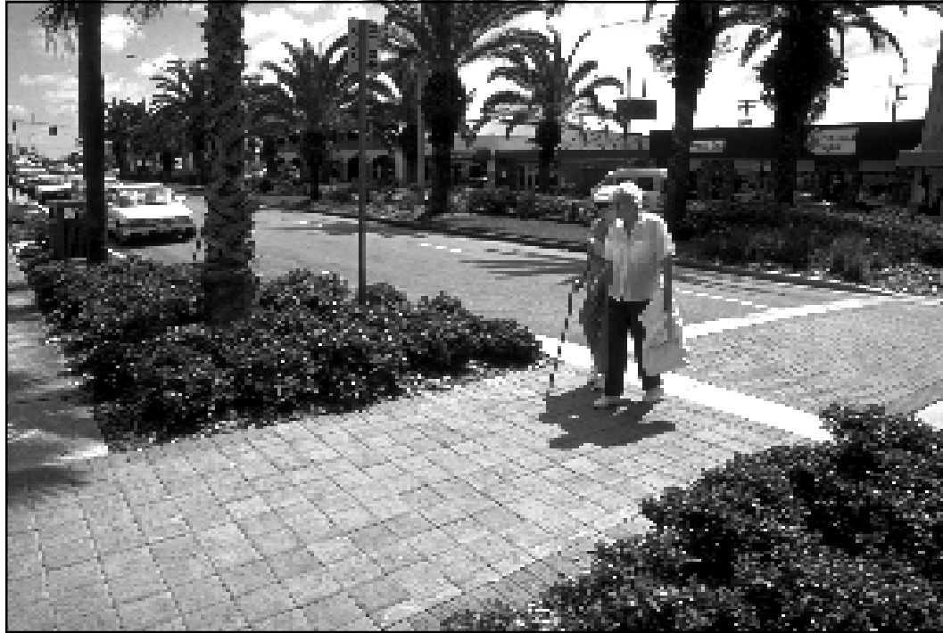
Figure 6-1. Properly built sidewalks are essential for increasing pedestrian comfort, mobility, accessibility, and safety.
