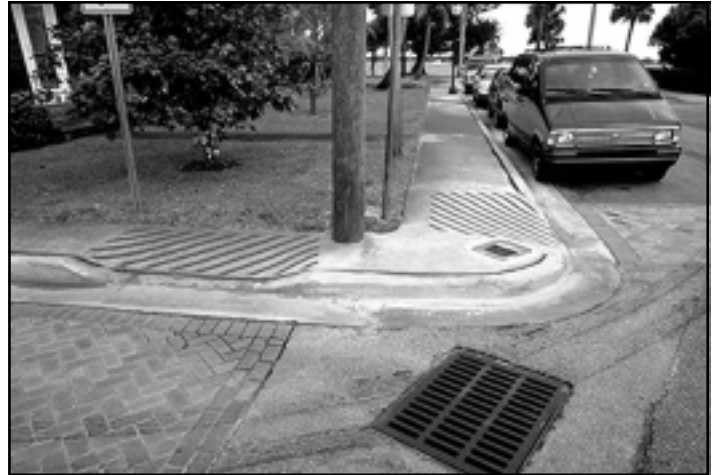
Figure 9-9. A tactile curb ramp.
