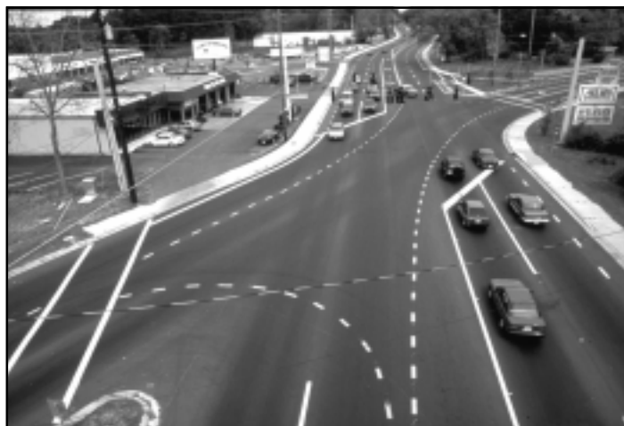
Figure 9-3. A crosswalk at a skewed intersection — there is a trade-off between making a 90-degree turn and staying close to the turning traffic.
