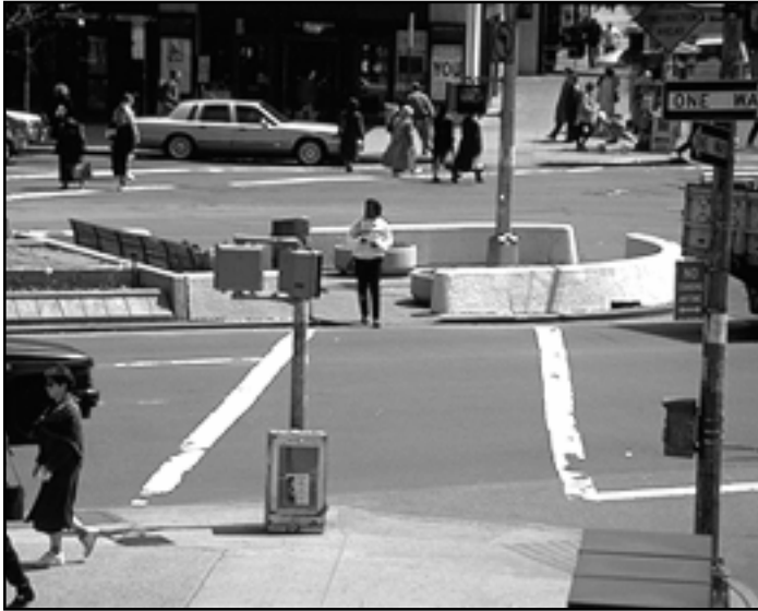
Figure 9-1. Properly designed crosswalks, curb ramps, and refuge islands can greatly enhance a pedestrian's ability to cross a street.
