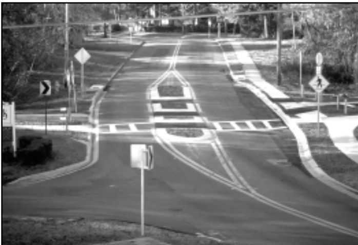
Figure 9-10. Refuge islands allow pedestrians to cross one direction of traffic, rest if necessary, and then cross the other direction of traffic.
