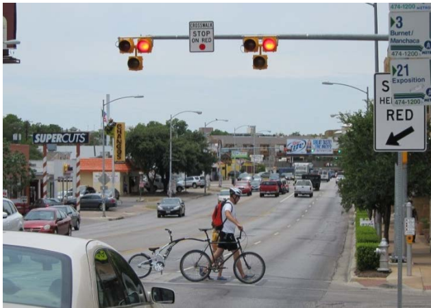
Example of a Pedestrian Hybrid Beacon treatment in Austin, Texas (source: TTI)
