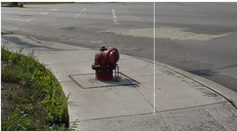
This fireplug is poorly located and obstructs sidewalk movements.
