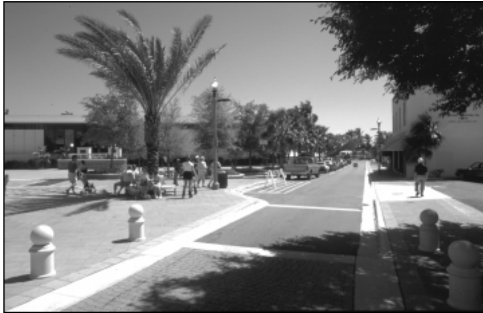
Figure 15-1. These medians and bulbouts calm traffic on this revitalized main street.
