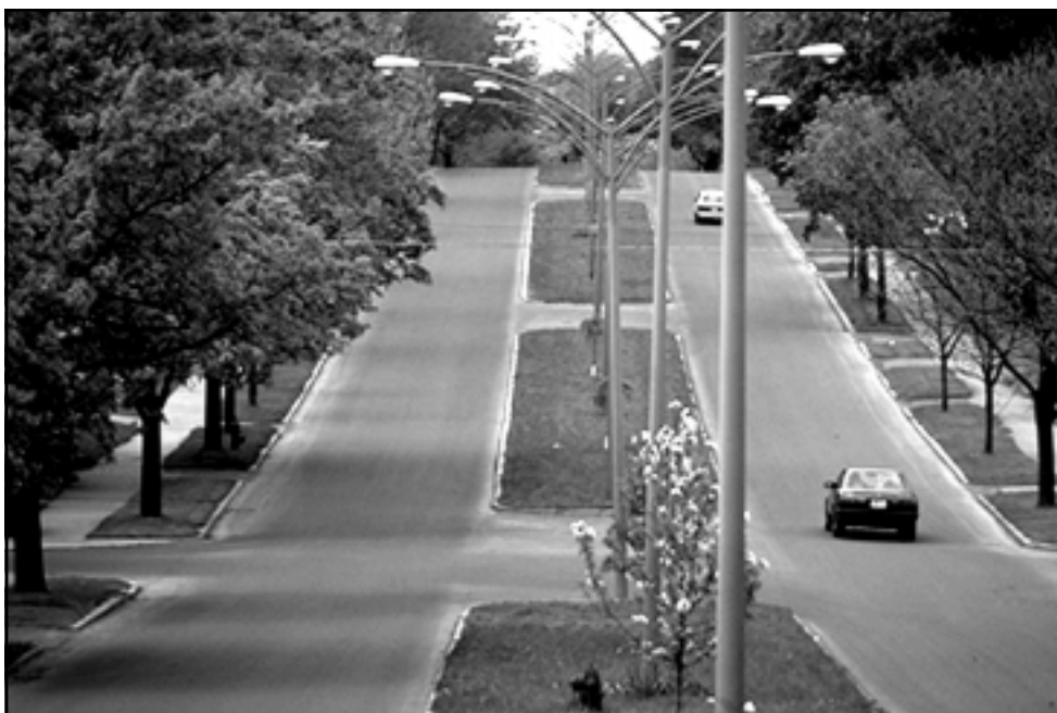
Figure 12-4. A raised median provides pedestrians a place to wait safely and to cross one direction of traffic at a time.
