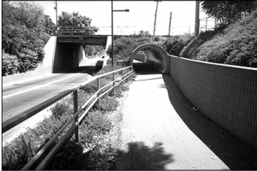
Figure 20-1. Grade-separated crossings improve pedestrian safety.
