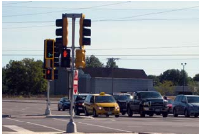
Median Pedestrian Refuge Area
