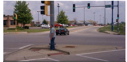
Right Turn Lane Corner Island
