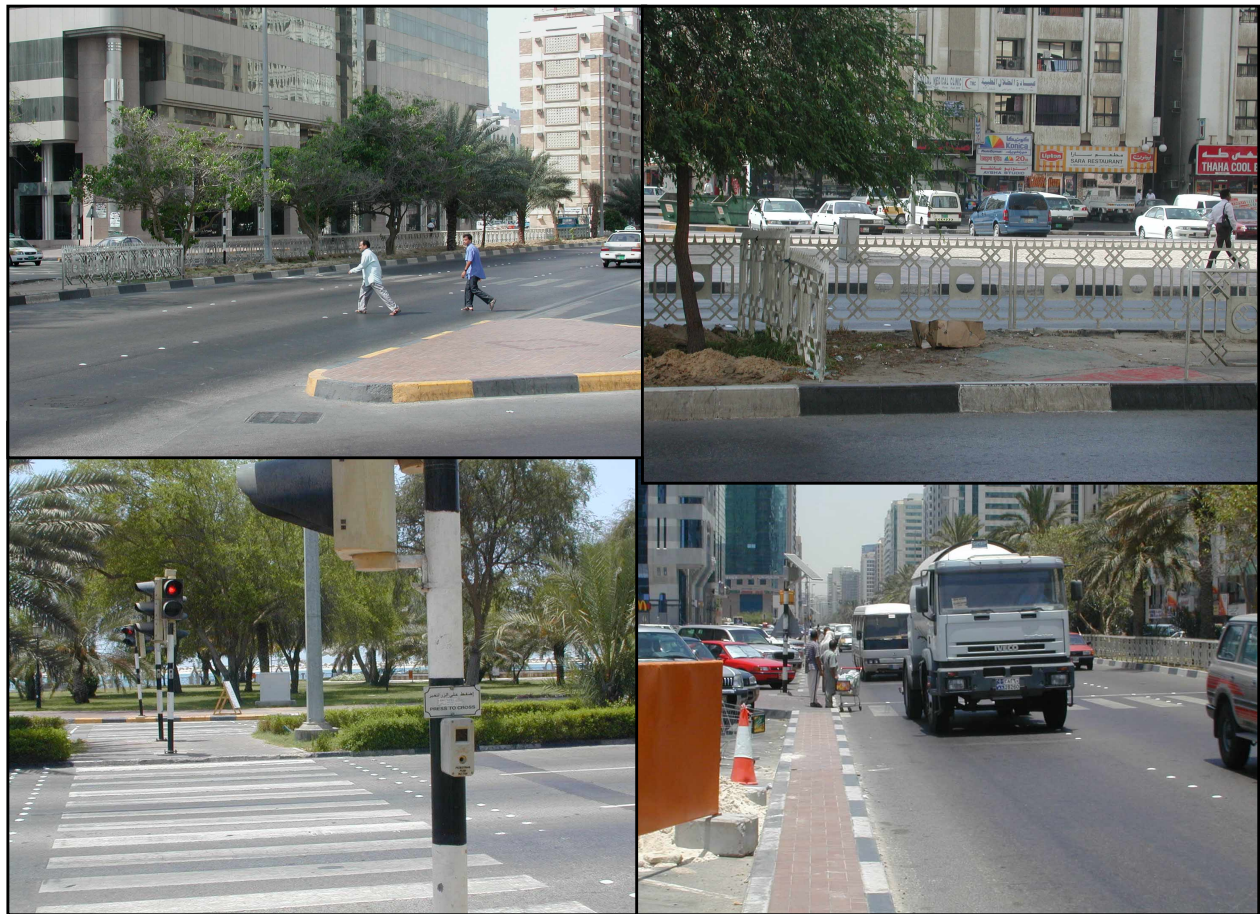
FIGURE 2 Examples of mid-block pedestrian crossings
