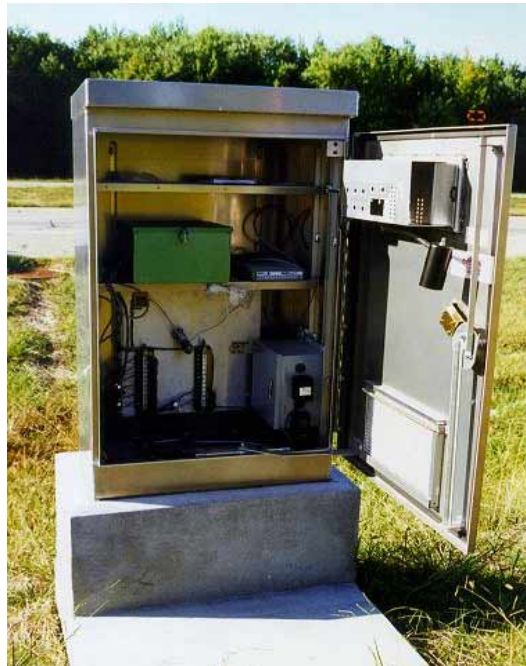
Figure 1 INDOT ATR (Automated Traffic Recorder) Permanent Count Station.
