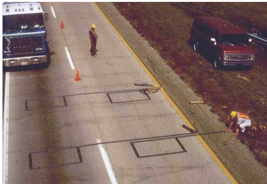
Figure 2 Temporary Sensors Installation
