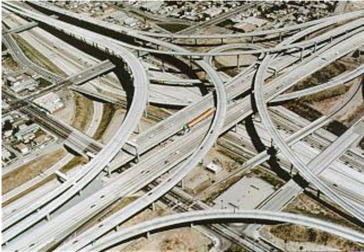
Interstate 105/Interstate 110 Interchange Los Angeles, California
