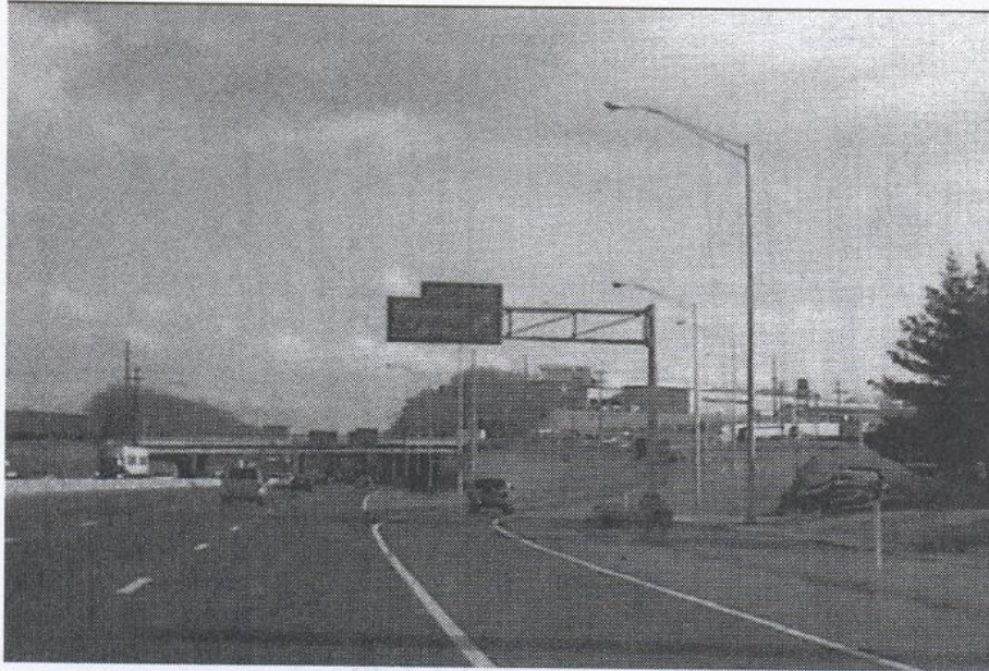
Figure 3-25. Two-Lane Exit—Undesirable Location.
