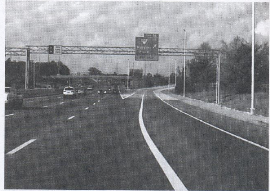
Figure 3-26. Two-Lane Exit—Preferable Design.
