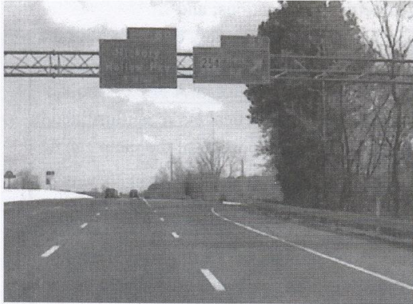
Figure 6-15. Decision Sight Distance—Undesirable Design.
