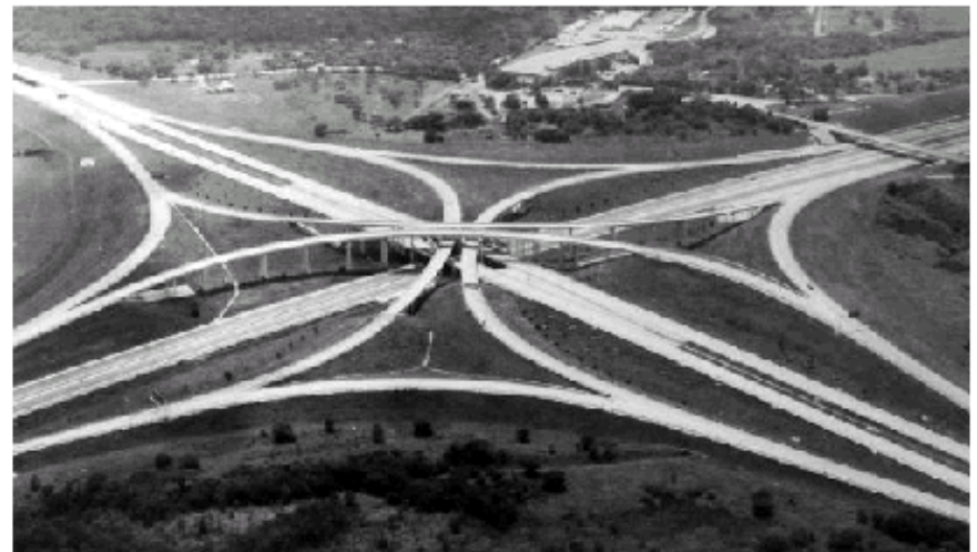
Exhibit 10-36. Four-Level Directional Interchange
