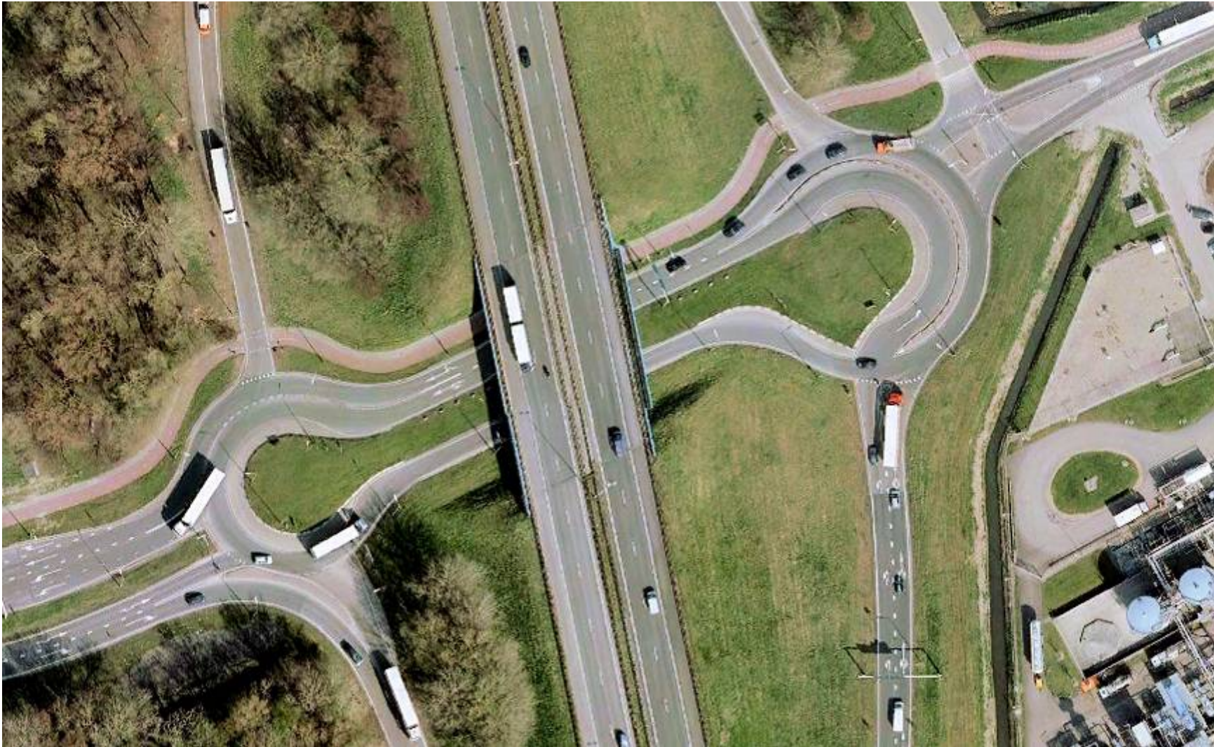
Maasdijk: Reconstruction of a diamond interchange
