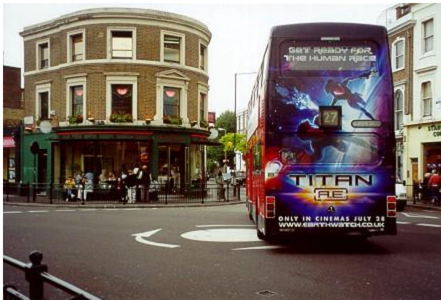
Mini-roundabout in Nottinghill Gate, London - Bus pass over center island (source: N.W. Garrick, July 2000)
