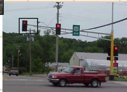
3-section Protected Left Turn Signal
