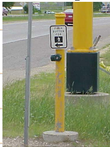
Pedestrian Push Button Station
