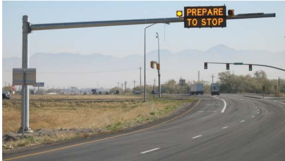
FIGURE 7.1.3 – OVERHEAD BLANK-OUT ADVANCED WARNING SIGNAL SIGN
