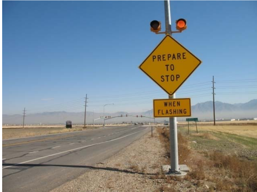
FIGURE 7.1.1 – SIDE MOUNTED ADVANCED WARNING SIGNAL
