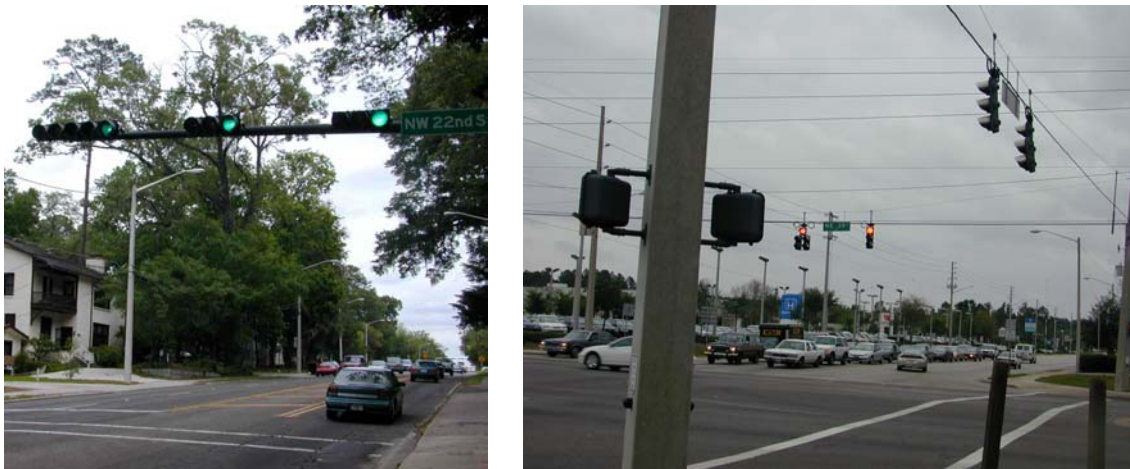
Figure 4-9. Typical Horizontal and Vertical Signal Installations.
