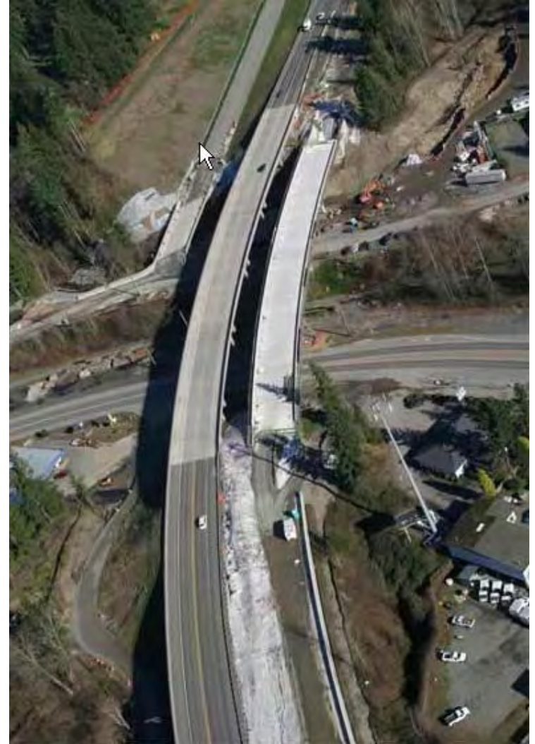
Bridge construction: SR 18 over SR 169
