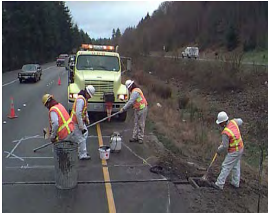
Electronic Crew installing Permanent Traffic Reporting site sensors
